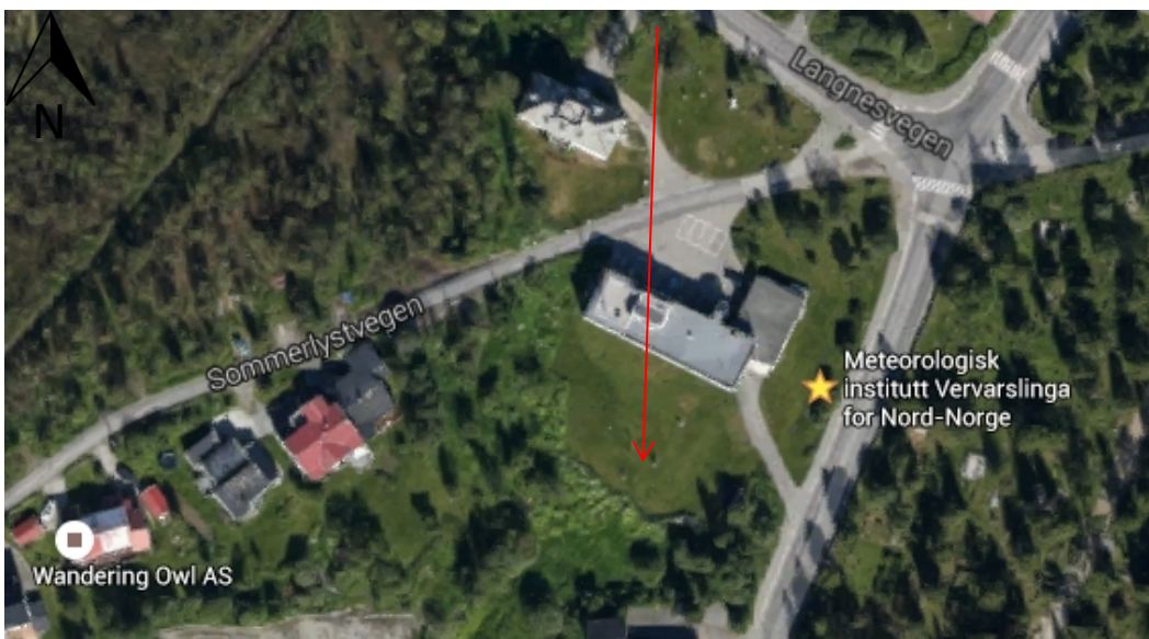
Figure 23: Aerial photo of 90450 Tromsø met station. The temperature screen marked red.
